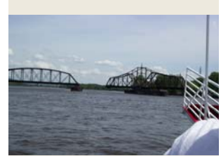
The Canadian Pacific railroad bridge.
